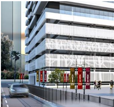
Perforated metal screens at podium parking
