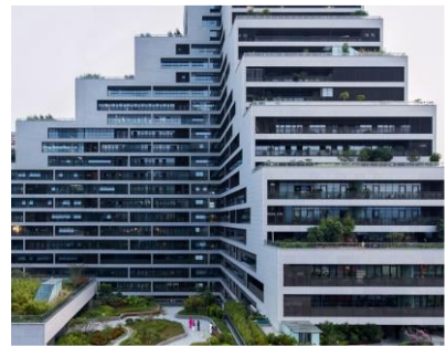
Segmented balcony facing waterfront
