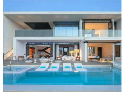
Residential glazed balcony
