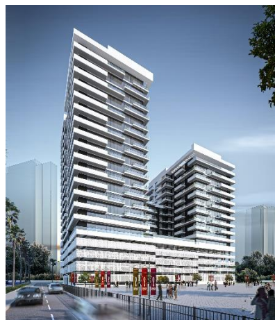
Mid-rise and tower with the same facade detail - legibility - with a clear separation of volumes.
