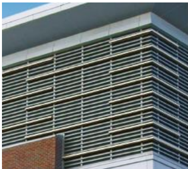
Roof tops technical feature covered with Screens as part of façade treatment
