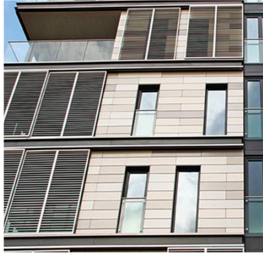
Screening as part of building facade
