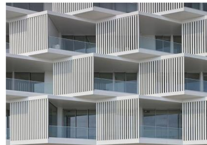
Shading devices over windows
