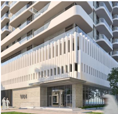
Vertical elements integrated in to the building facade
